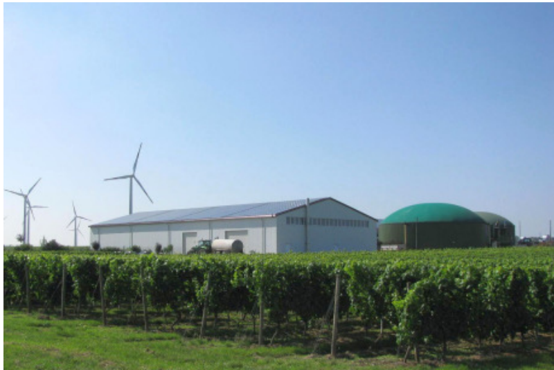
Abb. 48. Biogasanlage in Worms-Herrnsheim, © Stadt Worms.
