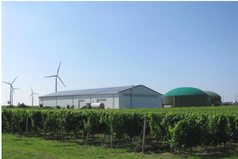
Abb. 48. Biogasanlage in Worms-Herrnsheim, © Stadt Worms.
